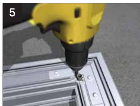
5 If supplied, fasten to each corner the tie bar drop rod fixing bracket to the underside of the lantern eaves beam.
